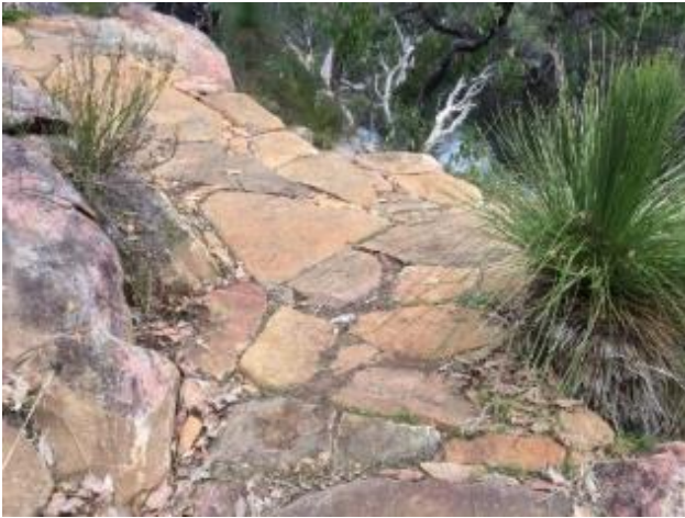
Constructed rock paving
