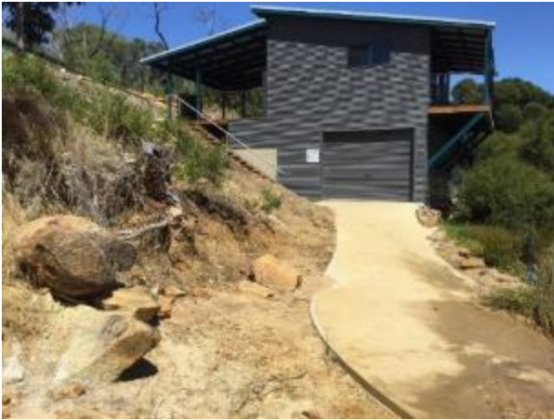
Degraded bare area at the Rowing Club
