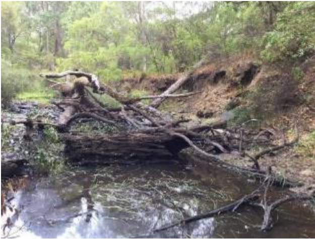
Bank erosion at Kilcarnup
