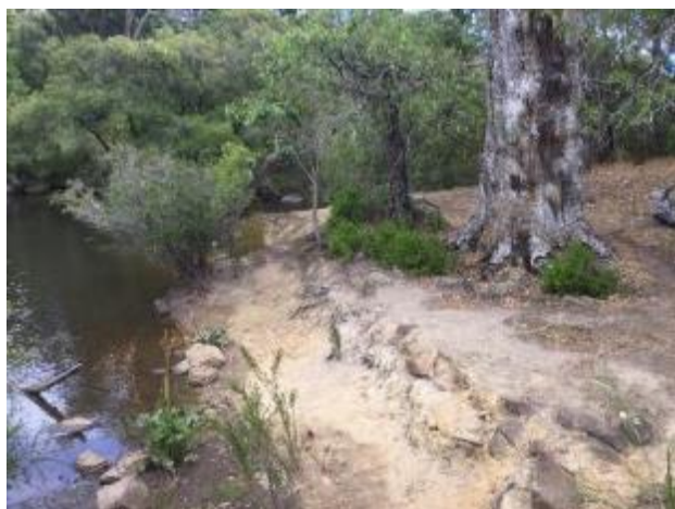
Erosion on the northern bank at the horseford
